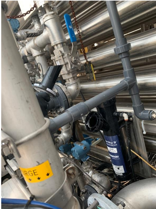
Figure 1 Turbidity sensor being removed from debubbler and measuring chamber
