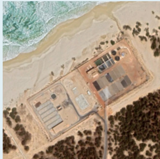
The Tivaouane Peulh FSTP in Dakar, Senegal, the proposed site for the commercial-scale J-OP
